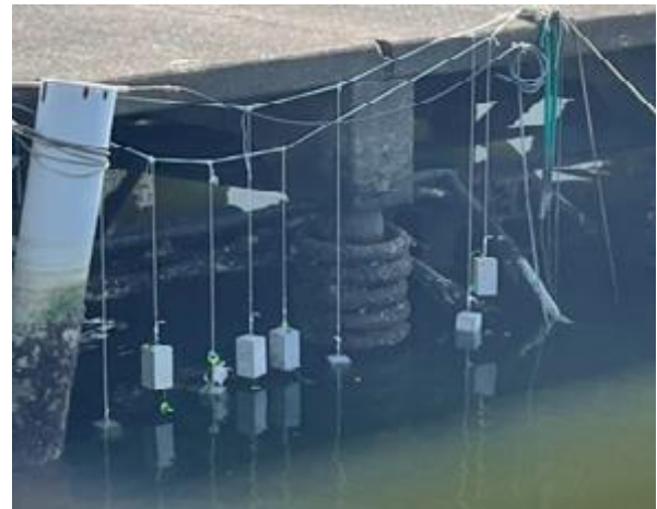
Fig. 3. Near Surface Condition in Zone B.
