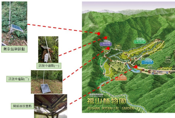
Fig. 7. Implementation of LoRa-support solar micro weather station, two repeat stations, and communication technology.
