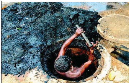
Fig.1: The above figure shows the basic way cleaning manholes i.e. man entering the manhole risking his life and subjecting him to many bacteria and viruses present in these sludge.
