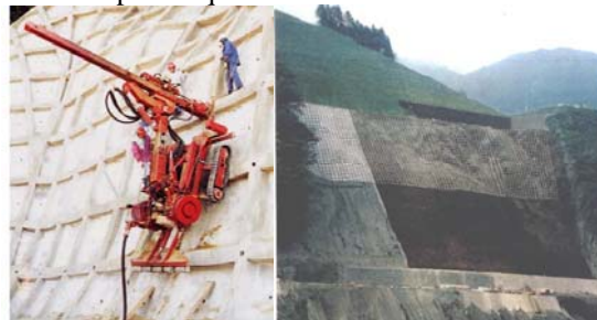
Figure.18: Conventional mechanized construction method on slopes
